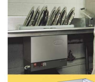
Individual controls (thermostat, high limit, low-water cut-off system, contactors) provide low cost repairs in the event of a failure.
